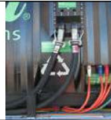
Data Power Cooling
