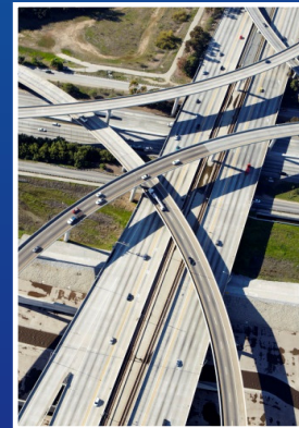
Smart Transport Infrastructure and vehicles
