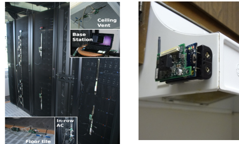
Green Home & Datacenter
